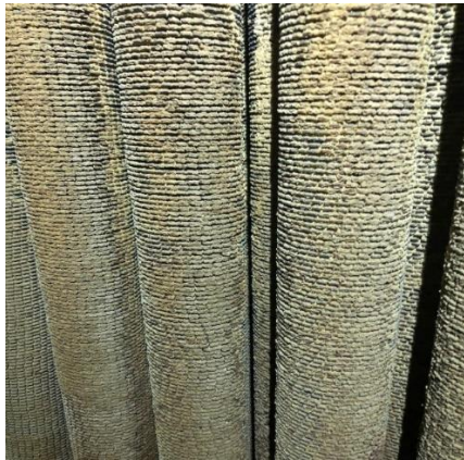
Tubes Before Cleaning
