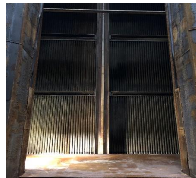
Boiler / stack floor completely clean
