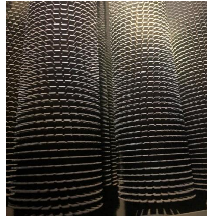
Tubes After Cleaning
