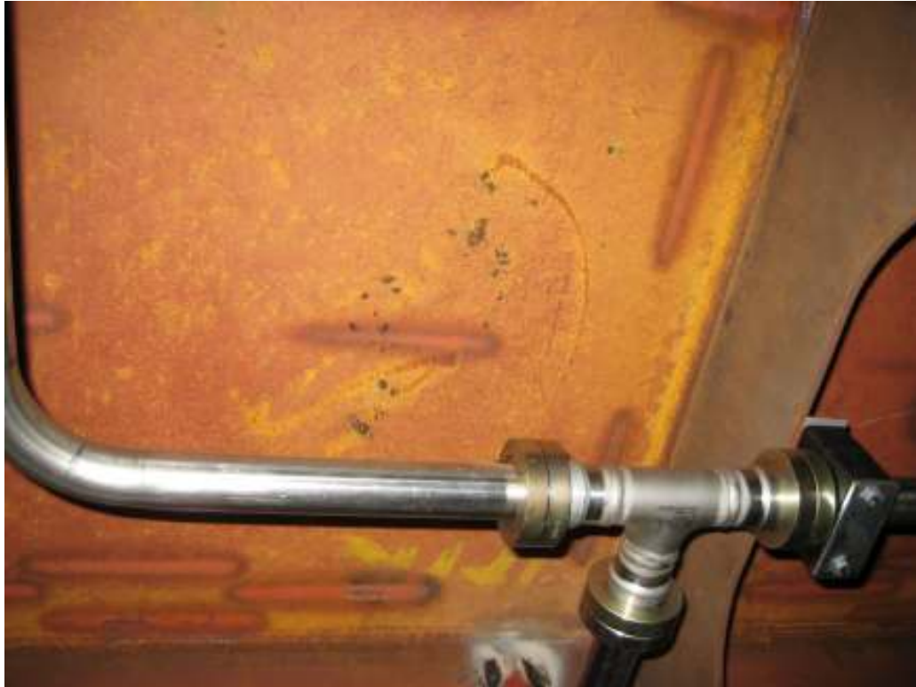
Photo 10 Before the CO 2 cleaning
