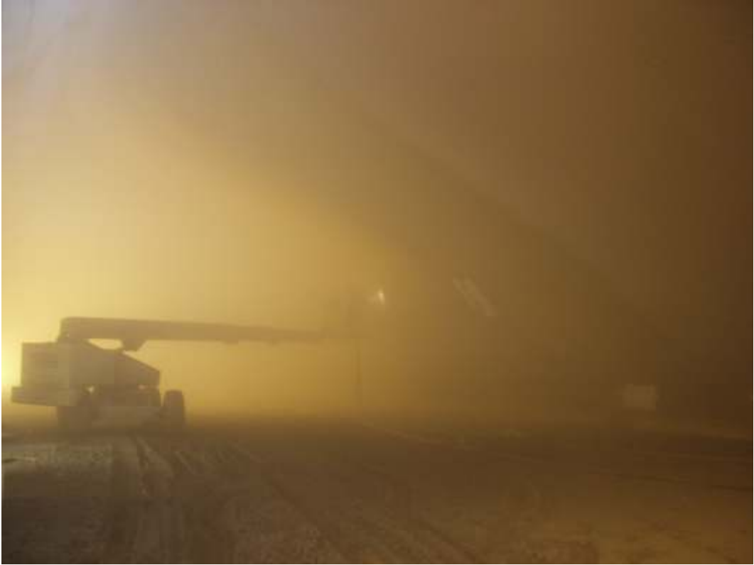
Photo 8: Dry blasting of under water hull for an Ice breaker coating system
