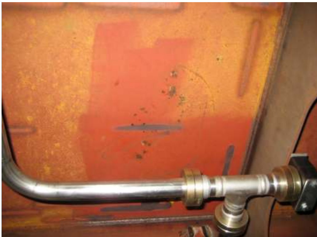
Photo 11 after the cleaning, even the burned shop primer has been fully removed
