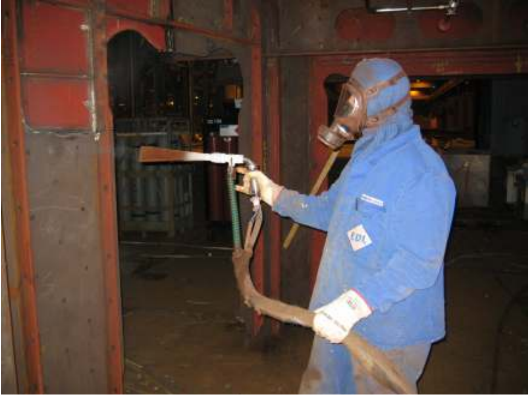
Photo 9: CO2 cleaning in progres
