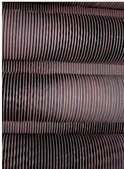
Before and after pictures of the cleaning, using tube spreading process
