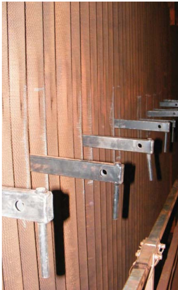
Tube spreading
